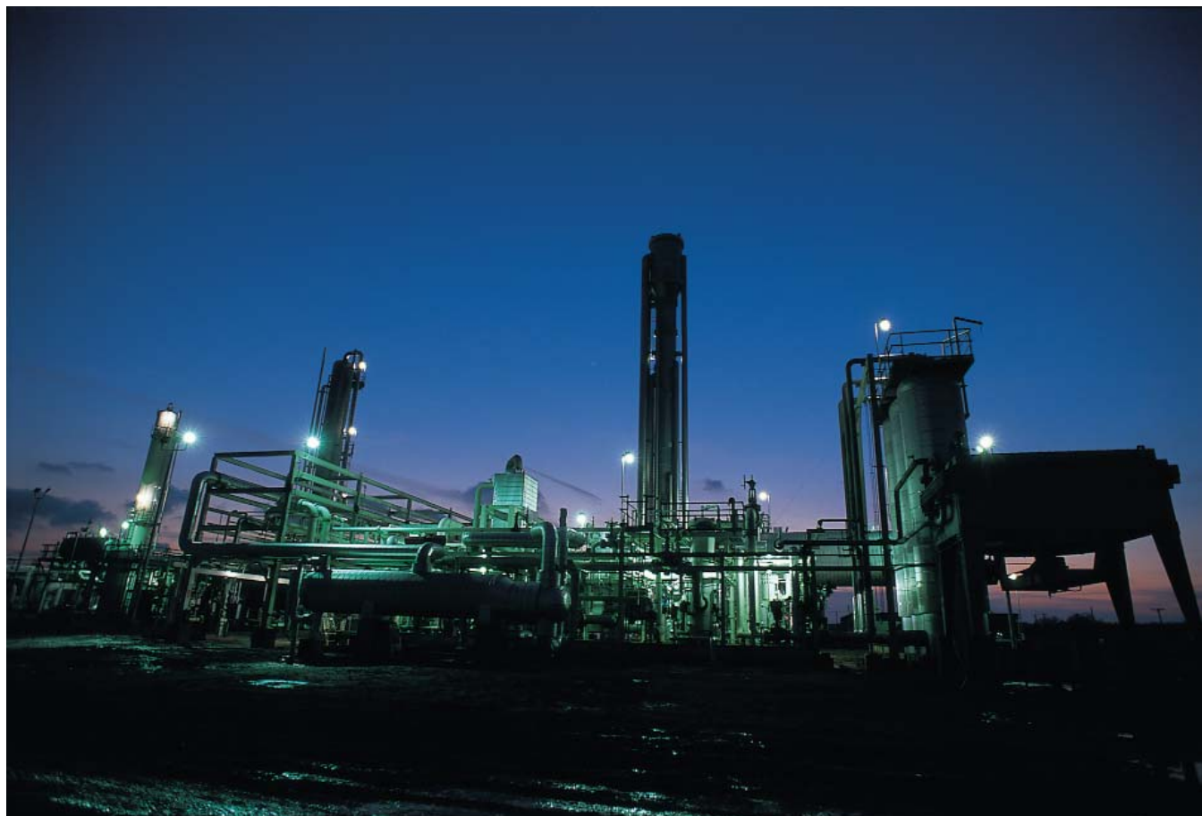
Devon's Bridgeport natural gas processing plant is one of the largest in the country, serving hundreds of gas wells in the rapidly expanding Barnett Shale field in north Texas. (Photo courtesy of Devon Energy)
